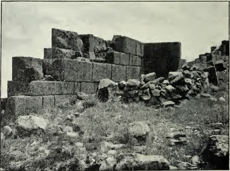
FIG. 243.—Bash Dagh, N. fort, curtain wall between polygonal and round bastions.
